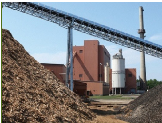
Black River Biomass Plant at Fort Drum NY Photo released by ReEnergy Holdings LLC
