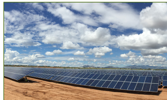
Fort Huachuca Solar Project ~1,000 panels mounted per day, September 2014
